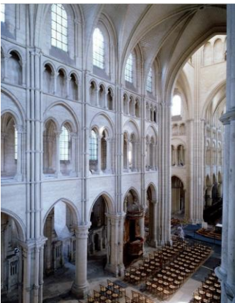
Interior view of Laon Cathedral
