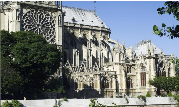
general view of choir with flying buttresses Notre Dame, Ile de Paris, Paris, France
