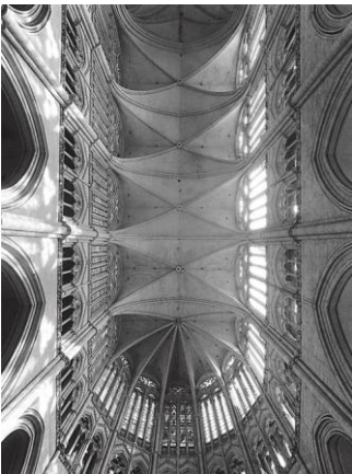
choir vaulting ( top ) and apse clerestory ( bottom ) of Amiens Cathedral
