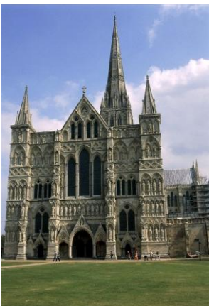
west façade of Salisbury Cathedral Salisbury, England 1220 - 1258 CE; west façade completed 1265 CE; spire completed ca. 1320 1330 CE
