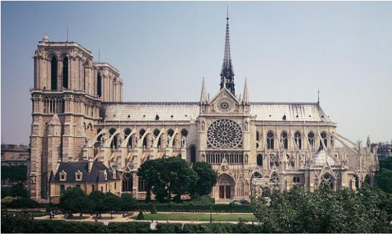
Notre-Dame; Ile-de-la-Cité, Paris, France Begun 1163 CE; nave and flying buttresses ca. 1180 - 1200 CE; remodeled after 1225 CE
