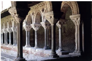
Cloister of Saint-Pierre Moissac, France ca. 1100 - 1115 CE limestone with marble relief panels piers approx. 6' high
