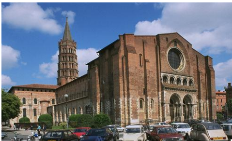
Saint-Sernin (view of façade)
